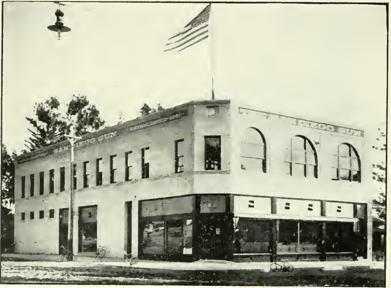
New home of the San Diego Sun Publishing Company, Seventh and B Streets, one of the most complete newspaper buildings in the United States.
